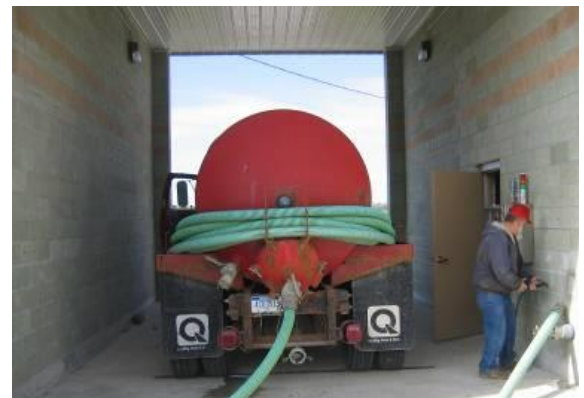
Unloading at septage receiving station. Septage bioreactor landfill reduces the cost to treat septage and eliminates septage pollution.
