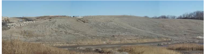
View of 7-acre full scale bioreactor showing green biogas extraction system. This bioreactor project produces enough landfill gas to power 800 homes or roughly half of the landfill’s overall potential.
